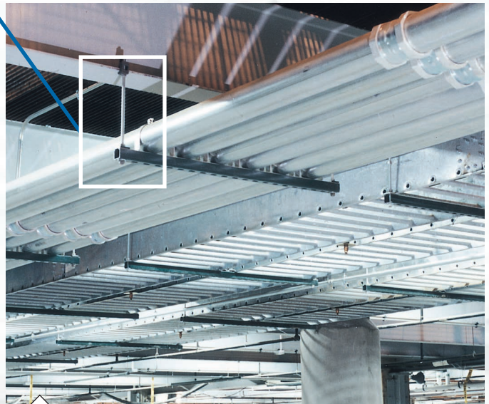
Beam clamp accepts standard threaded rod.
